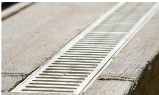
ADA-compliant polymer grate installed flush at court edge
