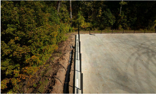
240-foot Swift drain HDPE run along the court perimeter — Renbrook School
