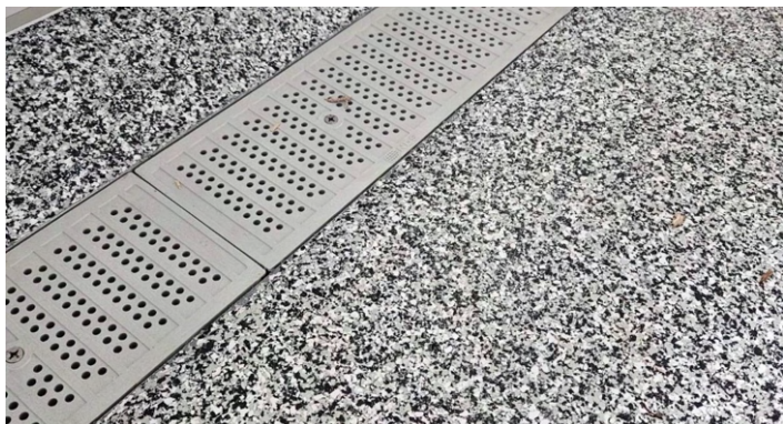
Swift drain paw-friendly grates installed in kennel floor — small circular openings protect claws and paws
