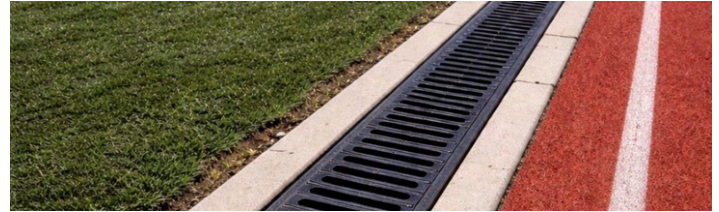
Swift Drain 6" pre-sloped trench drain installed along the inner edge of the running track — Tennessee high school athletic facility, 2021
